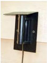
The outside sensor should ideally be placed on the east or north side of the house, away from direct sun light. The cover will help to keep water from staying on the sensor. The sensor can get wet, but it can be damaged from pressure washing or being sprayed with chemicals or paint.
