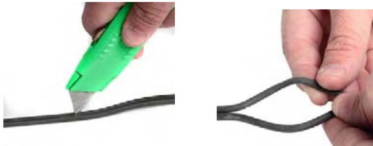
5. Take the fan connector wire that is provided. **The wires are already prepped and should not be cut off.** If you do the cut the wires, then you will need to strip 1 inch of wire insulation from fan connector wire and twist the copper back onto itself over the insulation on each side. This is important to make sure that there will be a proper connection.
