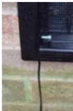
If running wire from the outside, the cable can easily be brought behind the fan at a corner of the grill.
